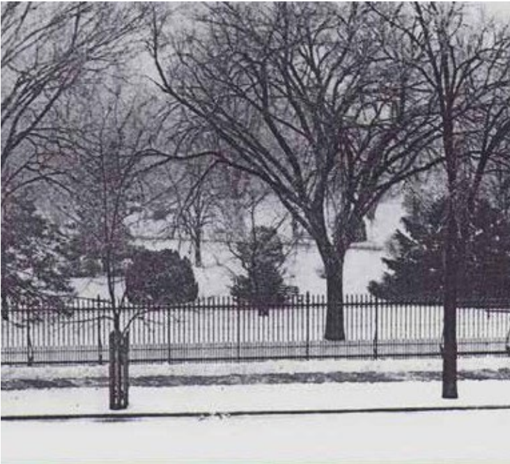
HISTORIC LAFAYETTE PARK FENCE
