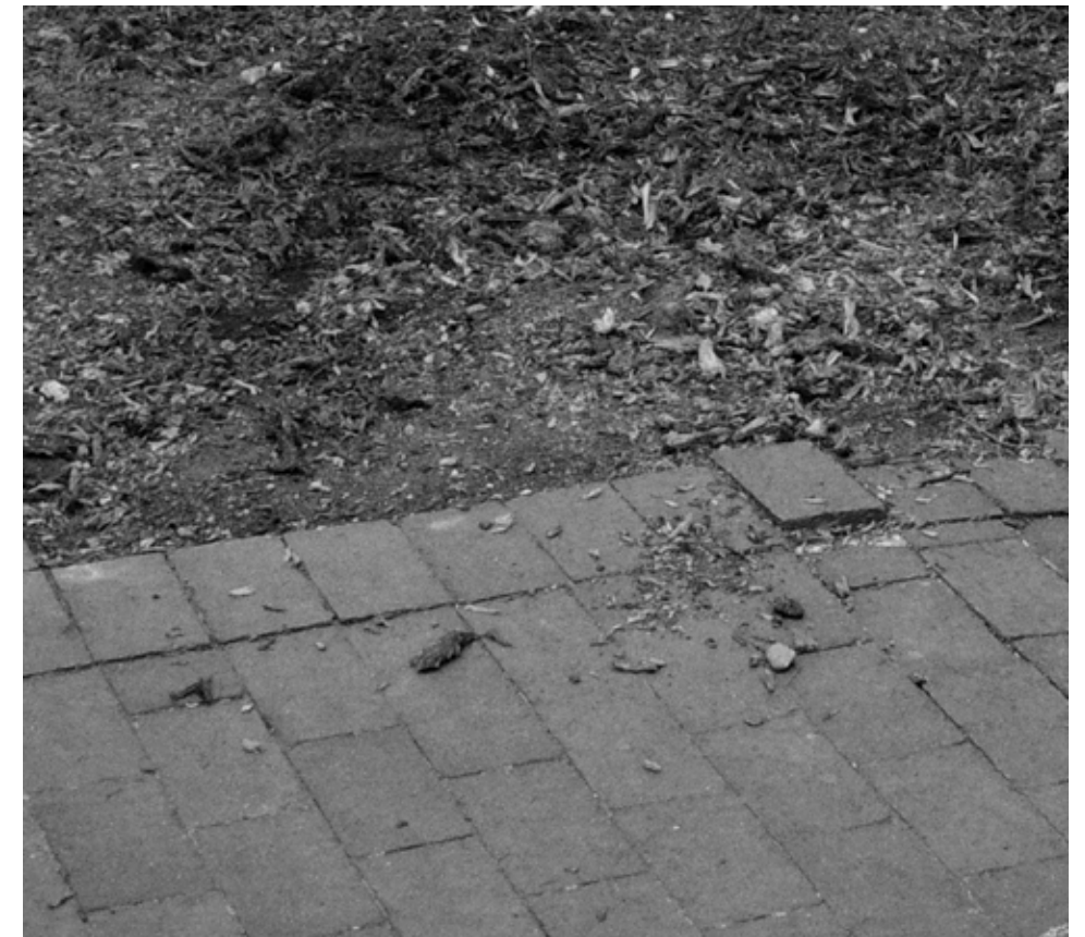
Site Visit Photos, 2026
