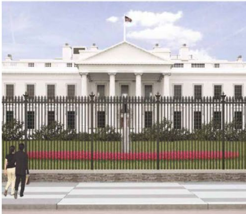
White House Fence
